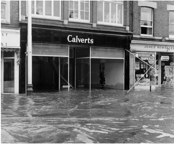
Calverts furniture shop, Station Rd – 1960
