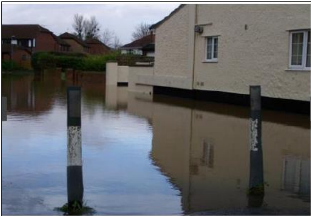
Figure 8 – Flooding outside Swingbridge House, Bathpool alongside the A38 in 2012 (Environment Agency)
