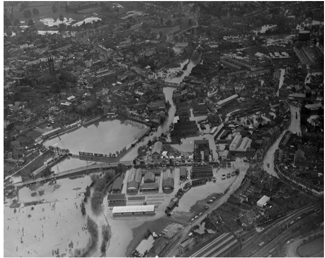
Aerial photo showing flood extent during 1968 event in Taunton
